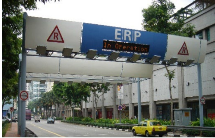
Figure 25 Example of fixed gantry with remote sensing technology. (Road toll in Singapore.)
